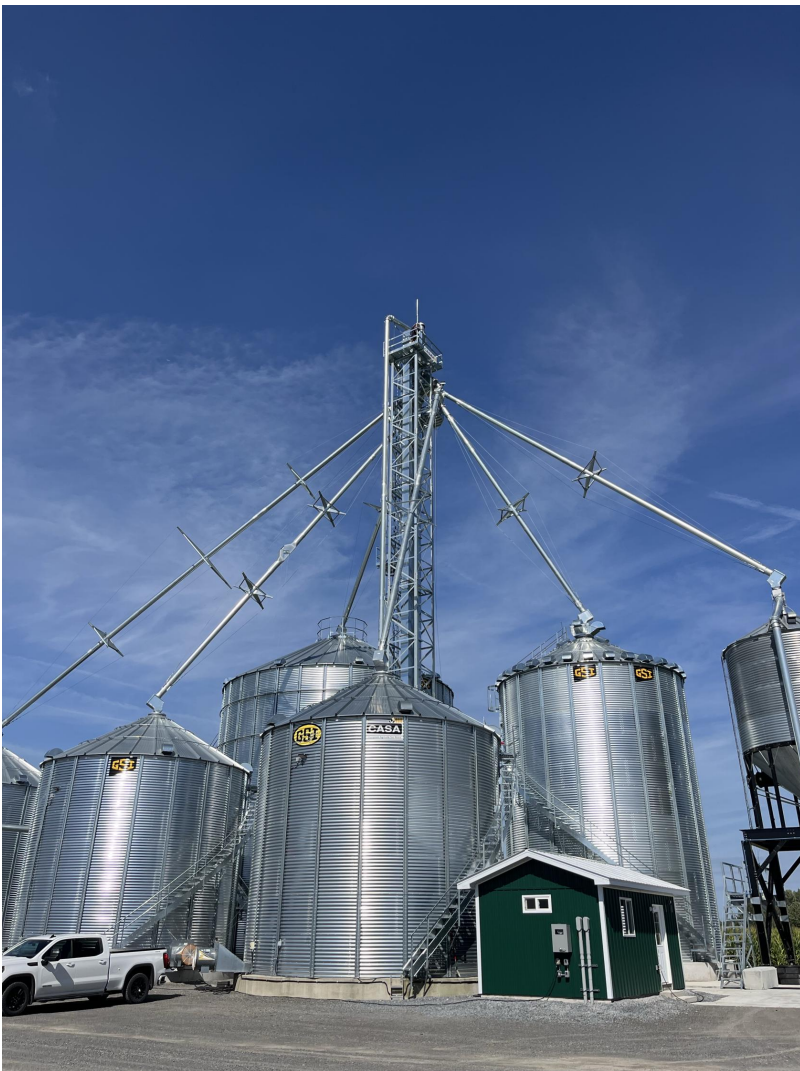
JockBrae Farm grain elevator and Ashton_GrainBin repeater site.
